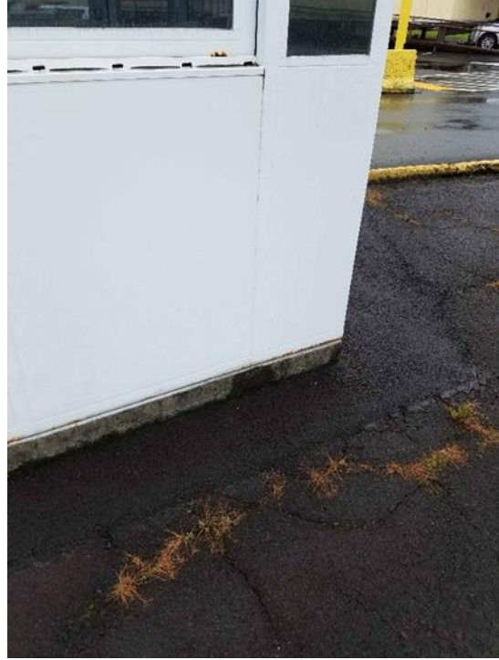
Existing guard shack on concrete base.
