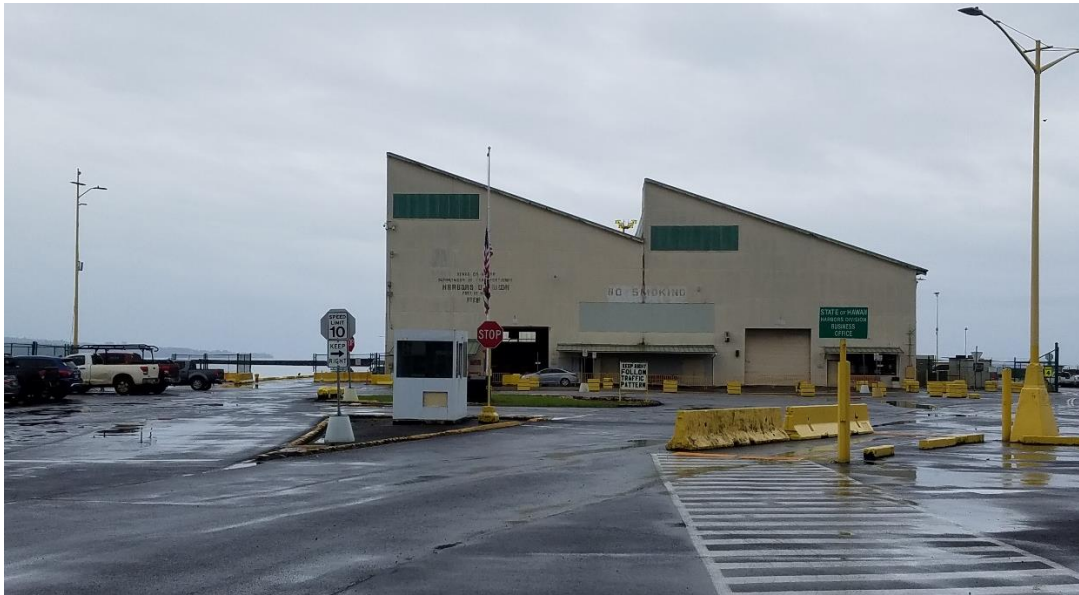
View from entrance driveway of existing guard shack.
